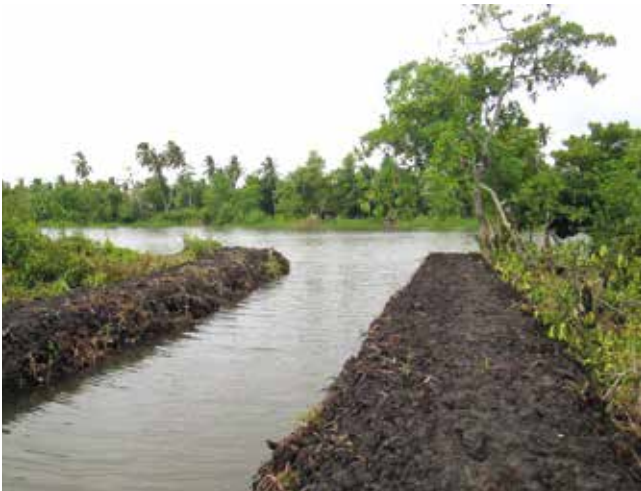
Left: Rehabilitated drainage channel.
